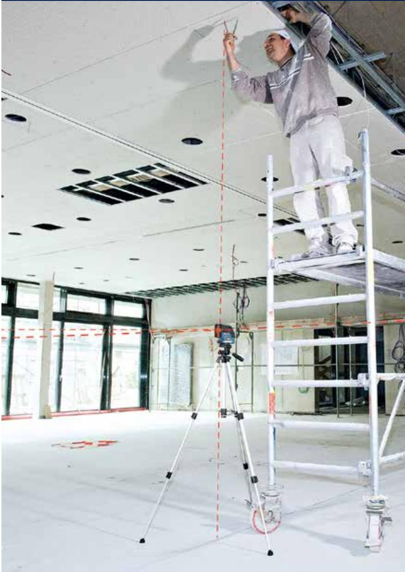
Bosch point alignment lasers precisely align, square and transfer points quickly and accurately, leaving hands free to get on with layout. Easily establish alignment, plumb, level and square. Highly visible and focused laser points ensure proper layout and installation on the jobsite.
